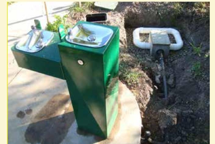
Right: Drinking fountain drains into a graywater system with a gravel infiltration basin.
